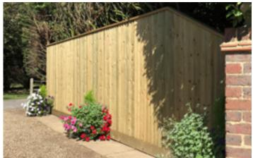
Traditional Featherboard is also known as Closeboard or Featheredge fencing. Supplied in kit form and constructed on site Traditional Featherboard is constructed with either 2 or 3 rails (depending on the height).
